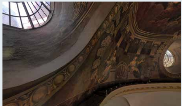
Laser scanning allows the dome's condition to be monitored in high definition including areas of cracking in the surface and painted decoration.
